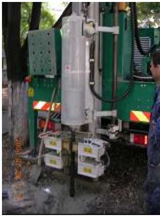
Figure 3: Standard Penetration equipment
