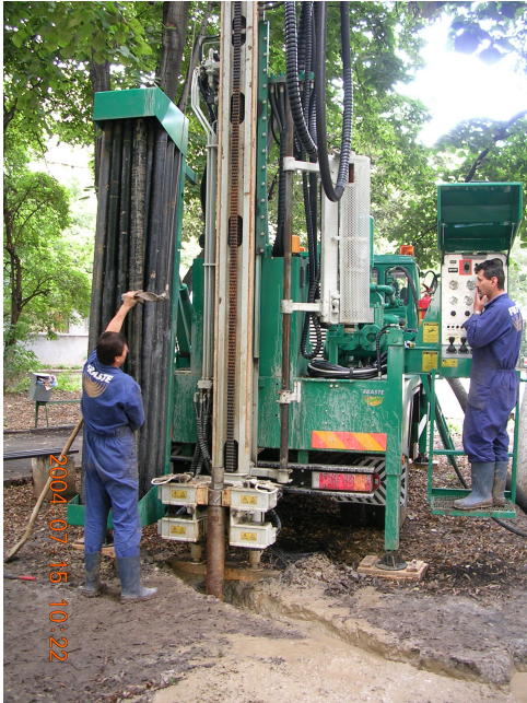
Figure 1: Drilling equipment (UTCB Tei site)
