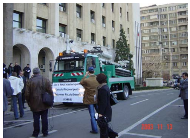
The truck with drilling equipment in front of the MTCT building
